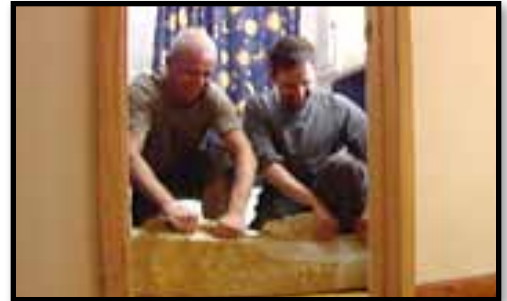
A. Removing the old linoleum floor.
