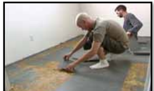
F. Laying cut tiles.
